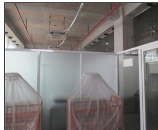
Photo of non-conformity Upper portion of segregation wall between child care room and medical room found in open condition.JPG
