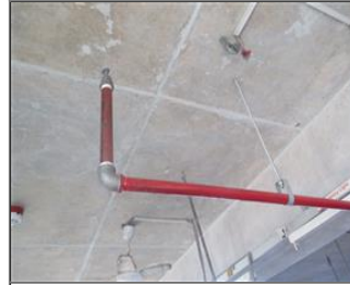
Photo of fire safety equipment Sprinkler system.JPG
